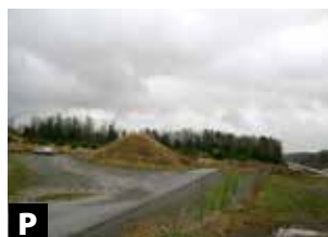
Main-lake parking area.
